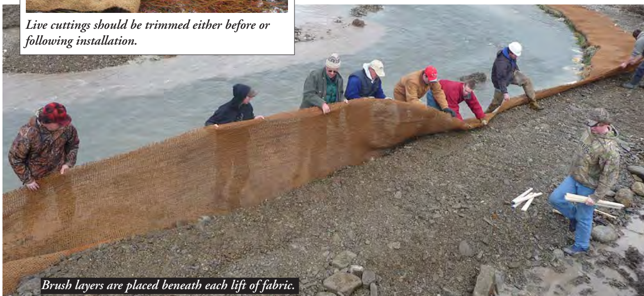
Brush layers have the best survival when placed near the water table or in moist soils. Irrigation may be required in droughty or coarse soils.
