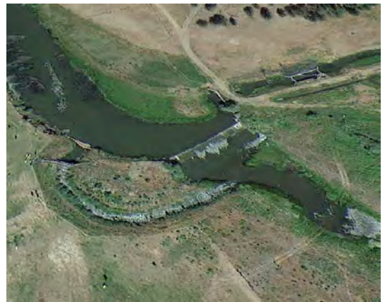
Engineered riffle bypass provides fish passage.
