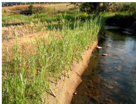
Willow cuttings work well planted through geotextile fabric if the basal end of the cutting can reach the water table. Irrigation is also useful to help establish new cuttings.
