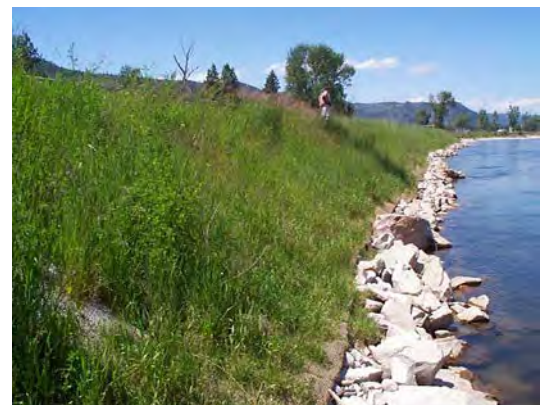
This site used rock to stabilize the toe, however, brush or woody debris would have been equally effective and preferred.
