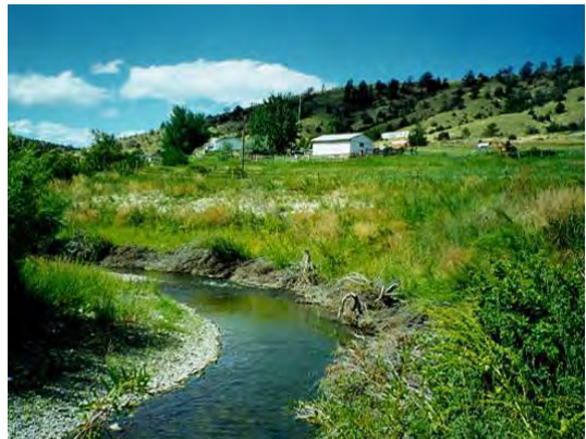
Restored bank using woody debris and sod transplants at the toe of the slope.
