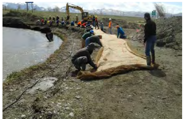
Geotextile bank treatments can be labor-intensive. Backfilled brush layer in place, ready for first soil lift.
