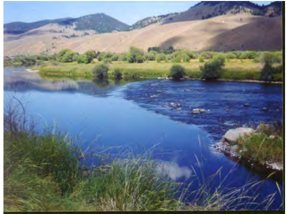
This weir has a relatively flat profile (without “cap” rocks) typical of an installation to check water at irrigation diversions. Caution: sediment transport can be reduced, causing channel instability in high bedload rivers.
