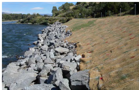
An engineered rip-rap bank provides a high degree of protection, but diminishes natural river and aesthetic values. These can be enhanced by incorporating vegetation above high water mark.
