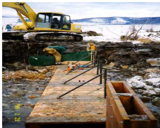
The flat floor and high drop of a pin and plank structure limits fish passage.
