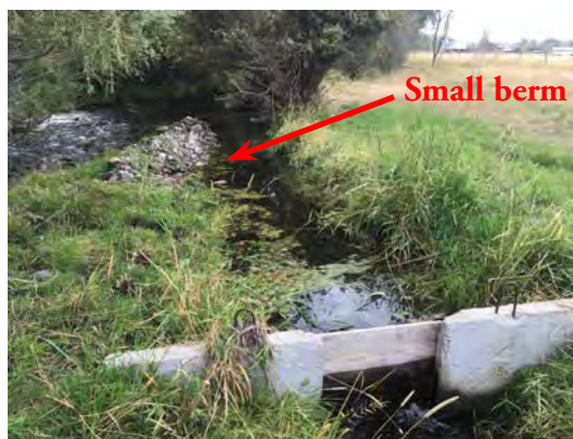
Small temporary berms may be appropriate in some locations as a low-impact alternative to permanent structures.
