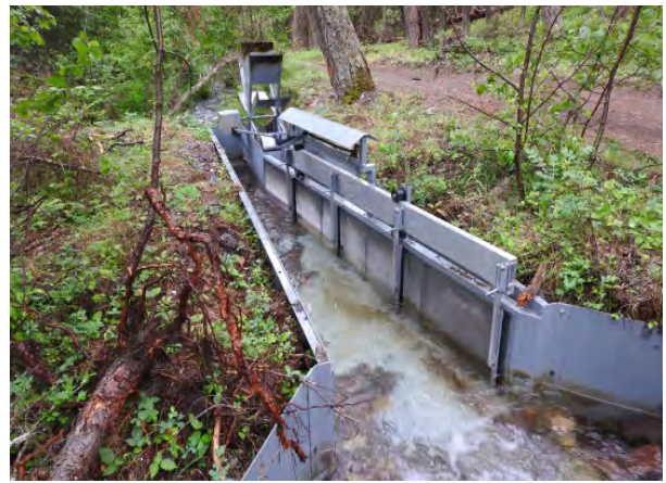
Fish screens on diversion structures prevent the loss of fish in irrigation ditches (entrainment)
