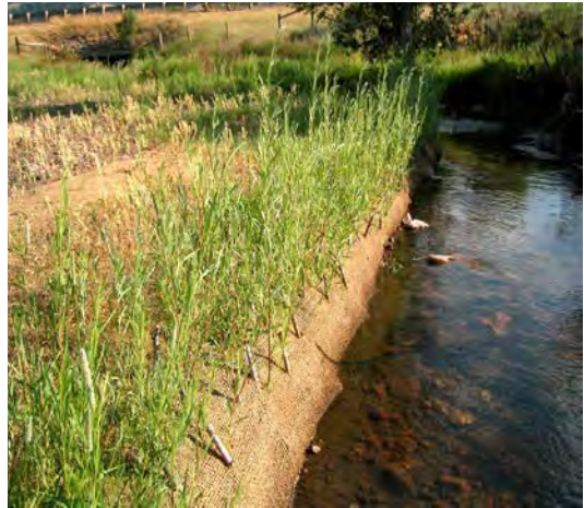
Creating an appropriate moisture regime is key to establishment of wetland and riparian species. Willow cuttings should be placed deep enough to intercept the water table.
