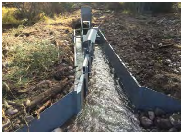
Vertical flat plate screens rely on paddle wheels to power the cleaning brushes. Bypass water returns young fish to the river channel.
