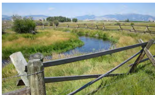
This meander has been restored to a more narrow, deeper form by channel shaping and bank sloping/sod mats.
