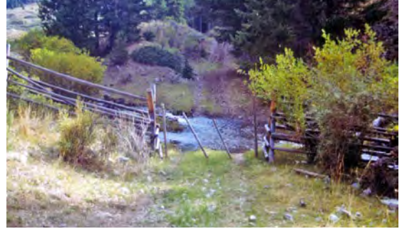
Stream crossings with long, steep downhill approaches often route sediments directly to the channel.
