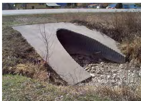
This arch pipe is sized to carry the predicted 25-year flow, but causes backwater at the 100-year flow.
