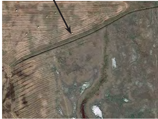
New drainage ditch
