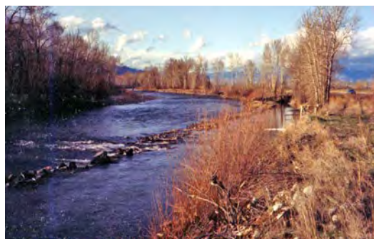
Gravel berms are essentially an extension of the ditch. Relocating the ditch entrance upstream may reduce the need for instream berms.
