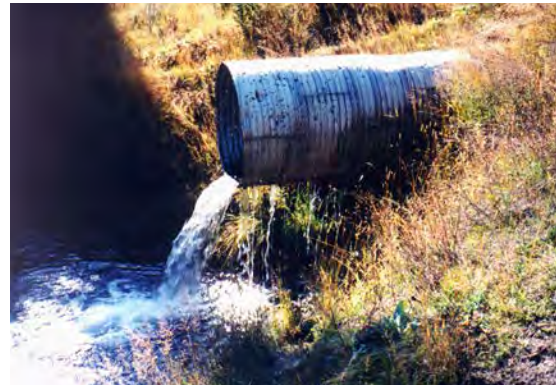
The shotgun (or perched outlet) culvert impedes fish passage, and can result from placing the culvert too high, or installing the culvert in a channel that has a tendency to downcut without grade control downstream of the outlet.
