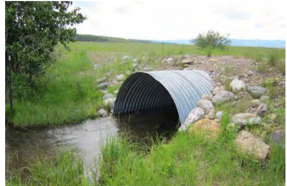
A well designed culvert allows for passage of flood events, and ideally, retains channel substrate material in the culvert to promote fish passage.
