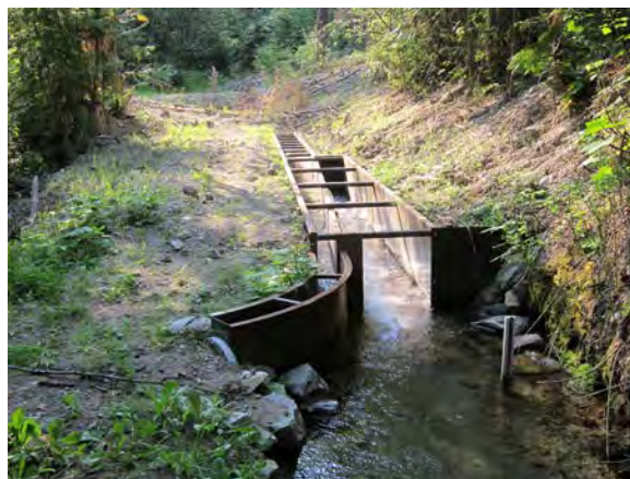
The screen entrance is in the background; foreground shows screened water on the right and bypass channel (fish return) on the left.
