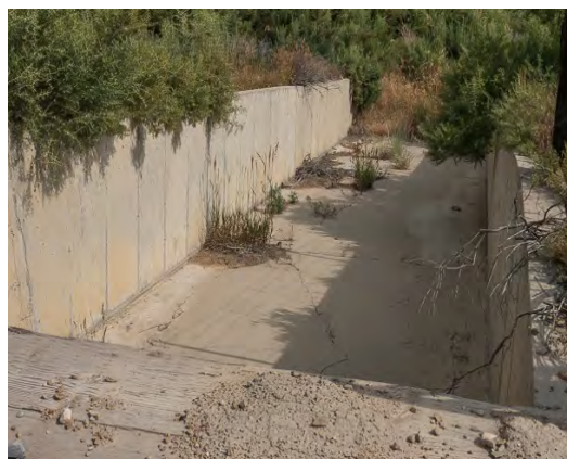
Dam spillway structures are commonly large rock or formed concrete and should be designed to withstand expected flood flows.
