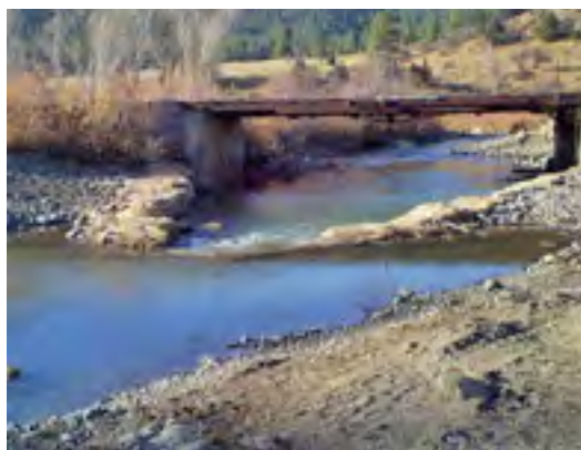
This crossvane weir is designed to control width-to-depth ratio alignment at a bridge cross section. Caution: sediment transport can be reduced causing channel instability in high bedload rivers.
