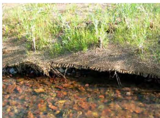
Biodegradable geotextiles can last 2 to 4 years while vegetation becomes established. Note, however, that the fabric in this photo has been abraded in the first year. Ultimately, all biodegradable fabric treatments rely on vegetation for long-term stability.
