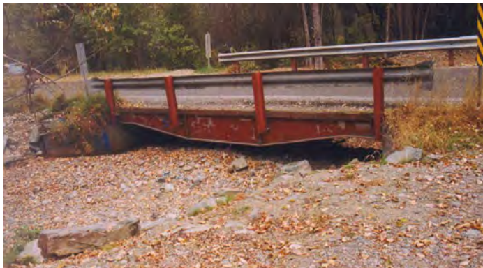
A low stringer in an aggrading channel does not leave much room for water. Note that the beam hangs low in the center and restricts peak flow capacity and debris passage.
