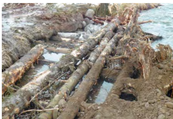
A robust toe protection technique relies on large woody debris to provide a high degree of scour protection.
