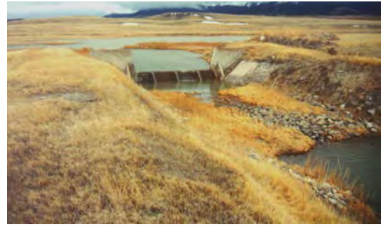
This large concrete structure functions as a cipoletti type weir.
