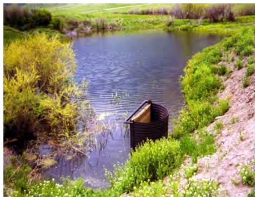
Canal checks are commonly used on small ponds to control water elevations. Canal checks and standpipe structures do not substitute for emergency spillways.
